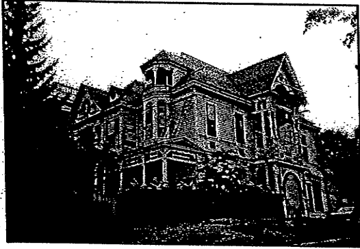
Left: M.O.S. Design, located at 600 Jefferson Ave, Scranton, before making façade renovations.
