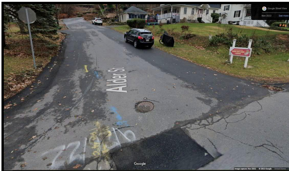
Photo 3.4.4 View looking up Alder Street towards the Marine Corps League Museum. Two stormwater inlets will be replaced along this section of the road.
