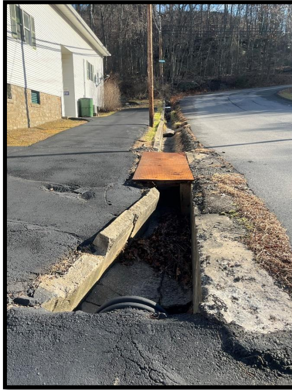
Photo 3.5.1 View looking up Beech Street from Wintermantle Avenue at the existing drainage ditch adjacent to the Discovery Montessori School.
