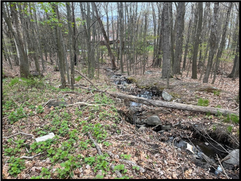
Photo 3.7.4 Stormwater discharges into this unmaintained drainage swale which had eroded and is filled with debris.
