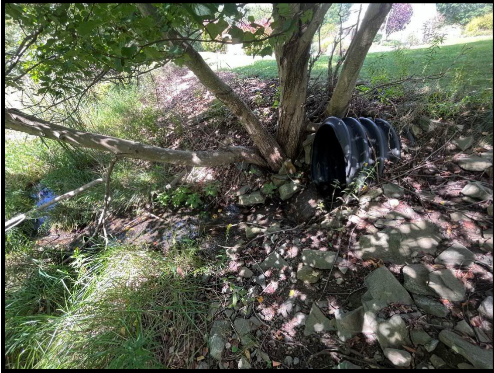
Photo 3.2.3 Existing discharge pipe from the drainage system along Cherry Street into the detention basin. It appears that only a fraction of the runoff from this street makes it into this basin.
