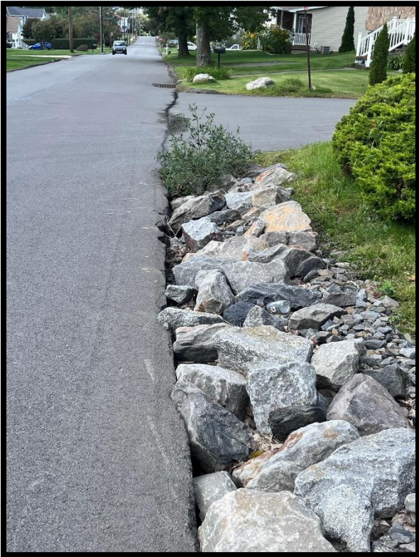
Photo 3.3.2 Excess rock within the East Elm Street drainage swale has significantly reduced its capacity which causes the swale to regularly overflow.
