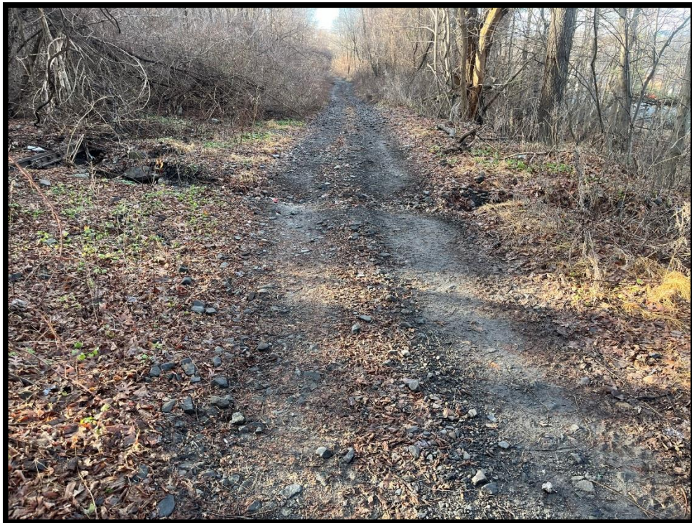
Photo 3.1.4 Concentrated flow of stormwater runoff from East Mountain has eroded ditches across the railroad grade.
