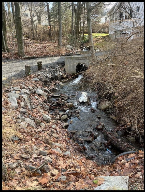
Photo 3.4.6 Further downstream, Mountain Lake Creek passes through this driveway culvert.
