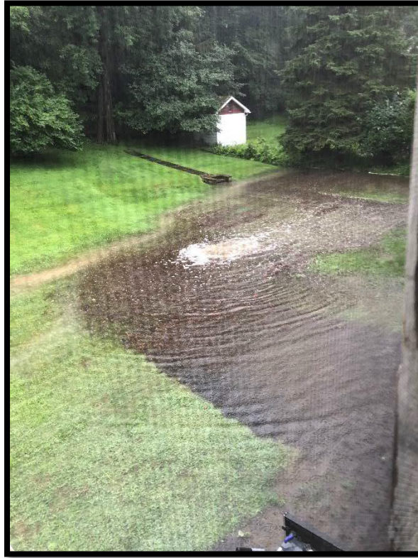
Photo 3.6.1 Homeowner's photo shows water discharging from a lawn grade during a flooding event. This indicates that the pipes in the lower portion of the drainage system must be blocked or collapsed.
