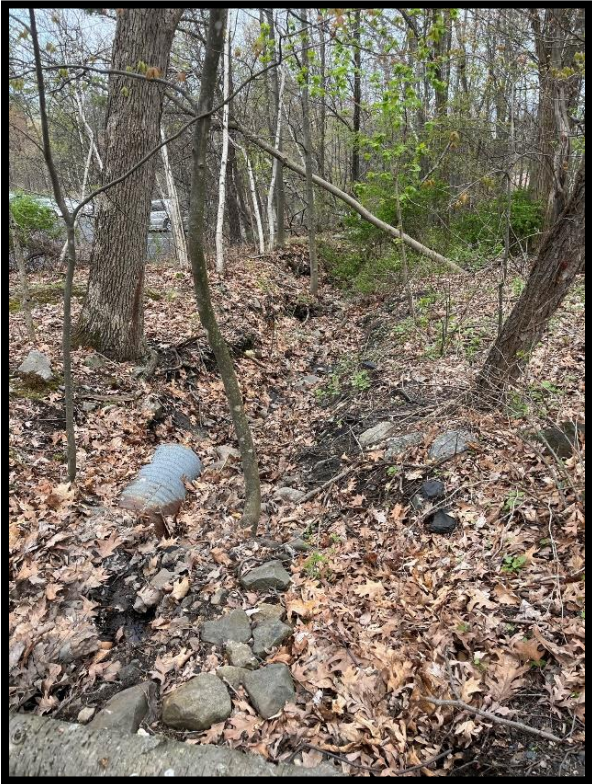
Photo 3.7.3 One of two stormwater discharges at the end of Ariel Street
