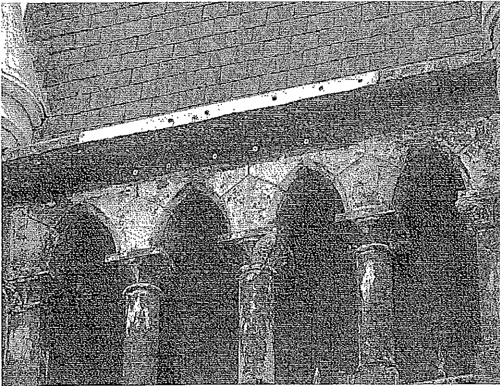
Photograph 30: Bird netting failure and infestation.
