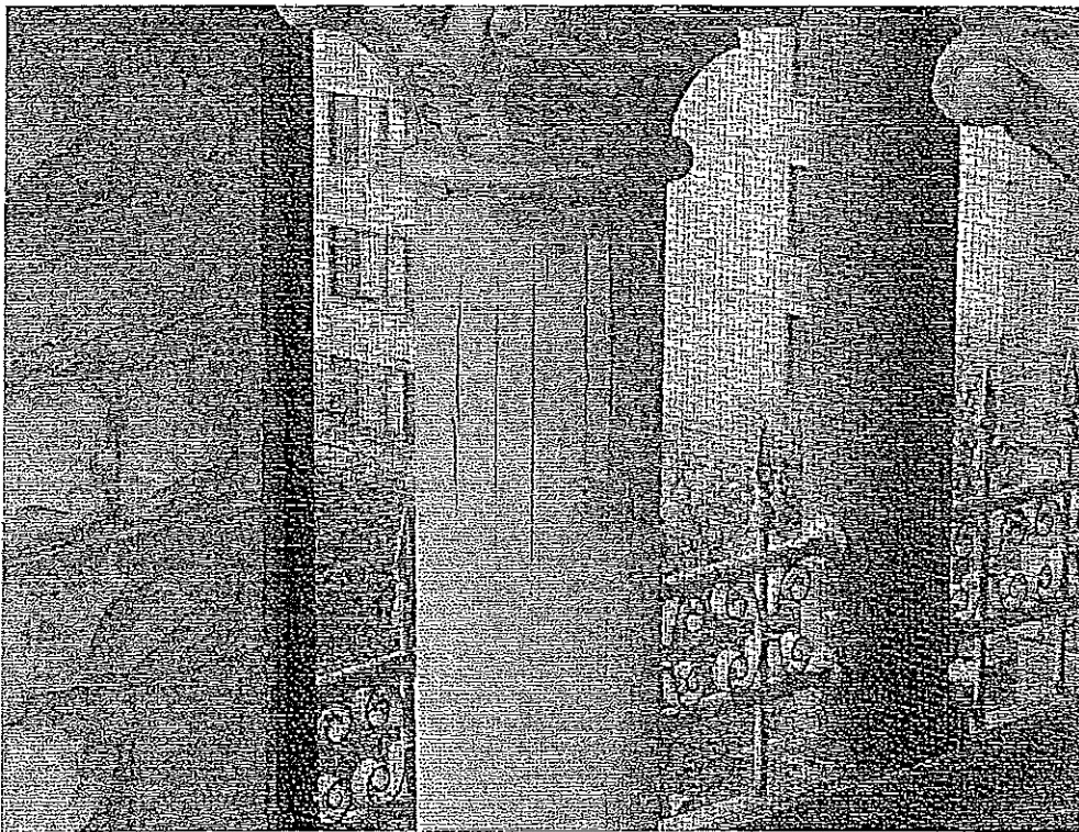
Photograph 14: Delaminated stone column shaft
