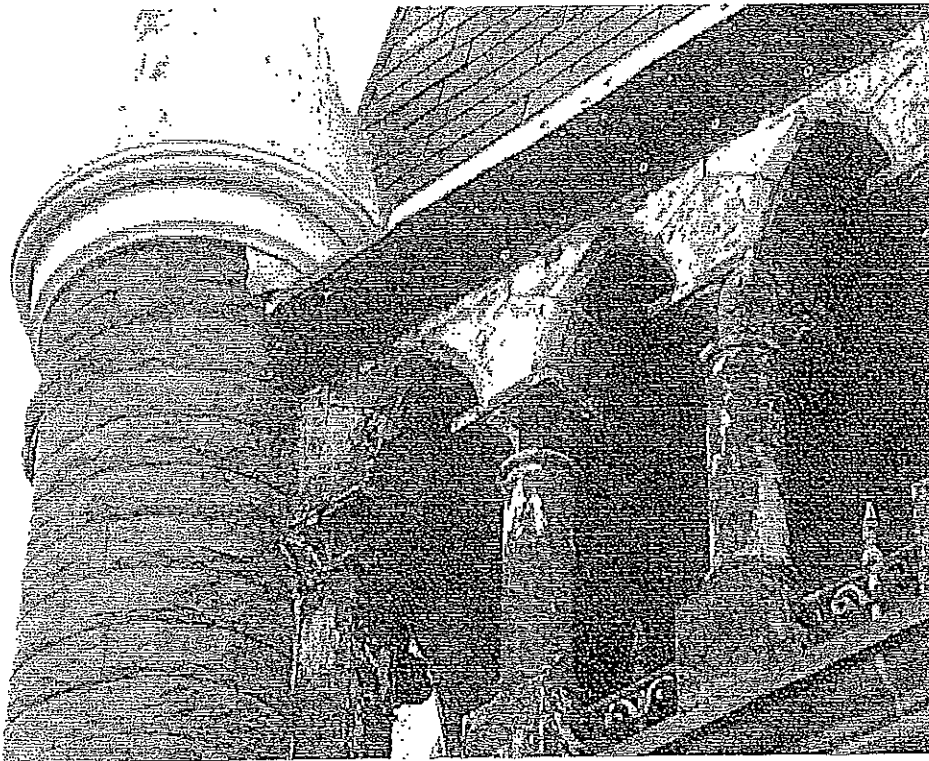
Photograph 28: Poor condition of cast iron and metal work.
