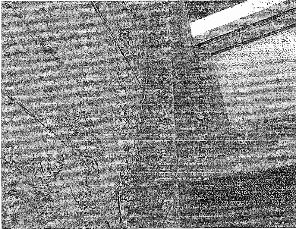
Photograph 31: Window perimeter sealant failure (typical).
