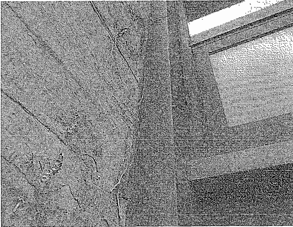
Photograph 31: Window perimeter sealant failure (typical).
