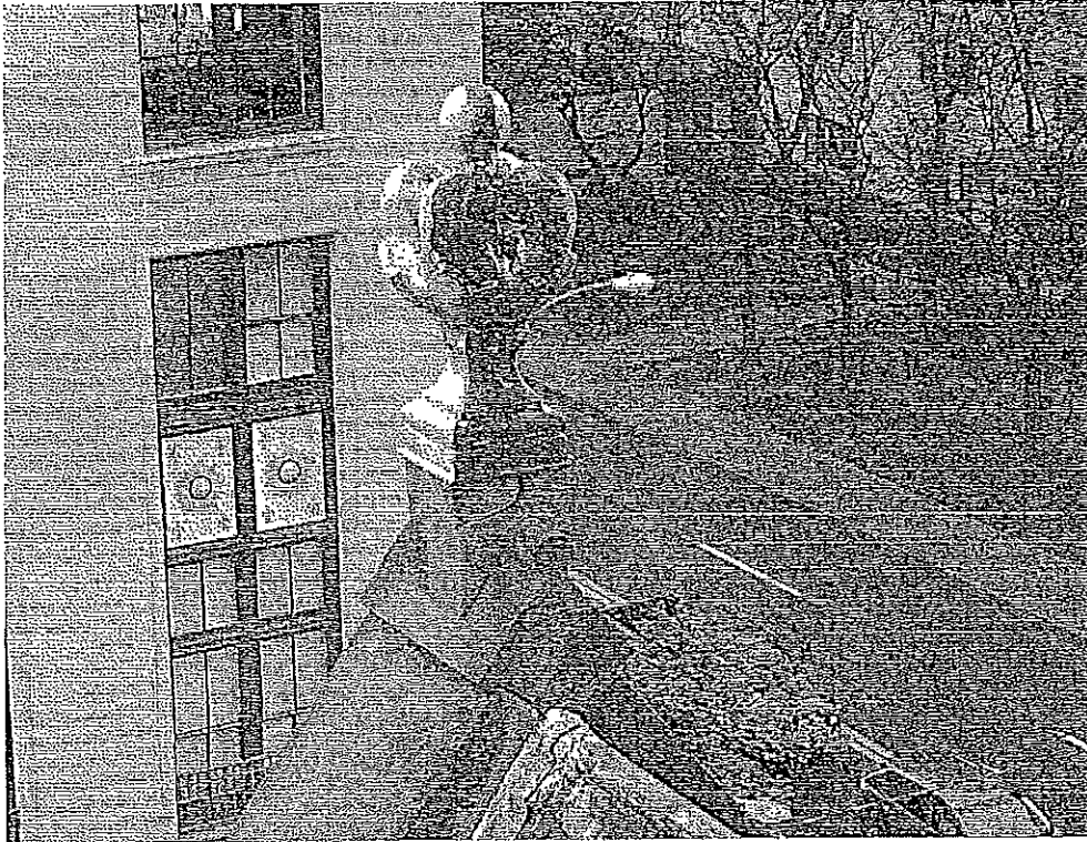
Photograph 23: Cracked stone finial base
