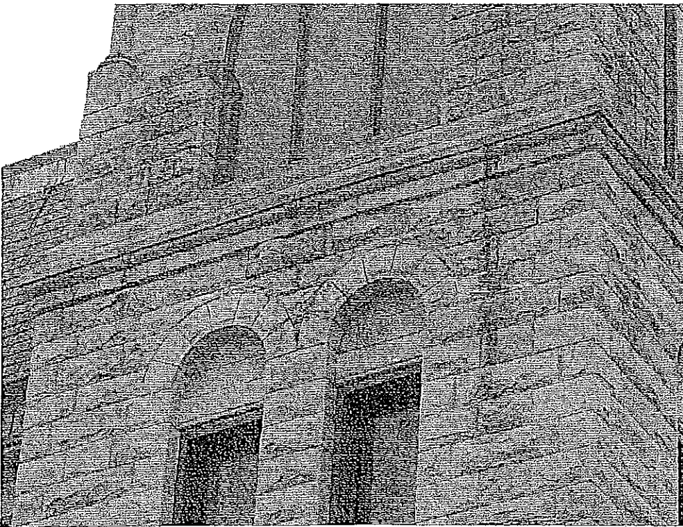
Photograph 10: Stone displacement and mortar joint deterioration allowing water infiltration
