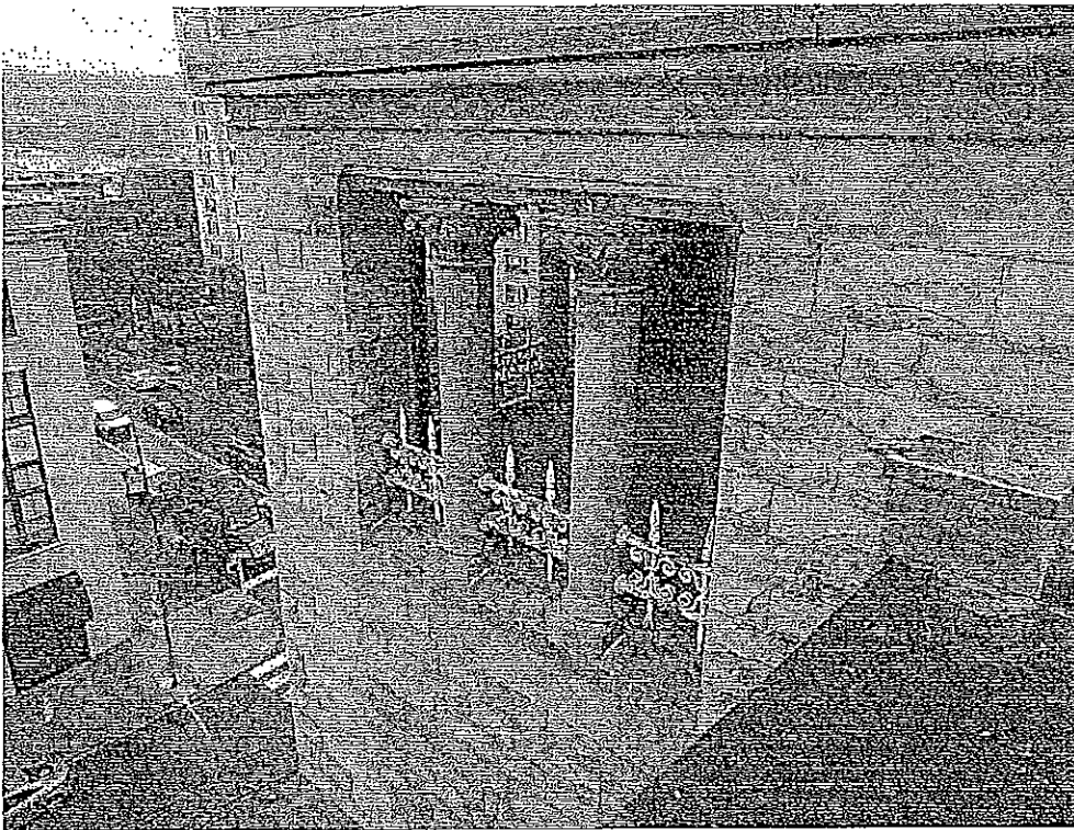
Photograph 16: Open tower level. Note also two different types of stone; rough cut ashlar units and smooth faced decorative units.
