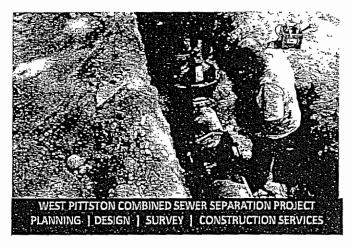
approximately 3,000 feet long was designed. Approximately 6,700 feet of collection storm sewers ranging in size from 12 inch to 36 inch diameter have been constructed throughout the drainage basin to collect and convey storm water into the main culvert. Approximately 16,000 lineal feet of sanitary sewage mains were constructed. New sanitary sewer laterals were installed in the streets and new manholes were constructed. The project was bid in 2009 and completed in 2012.
